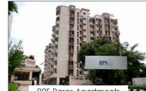
RPS Paras Apartments
